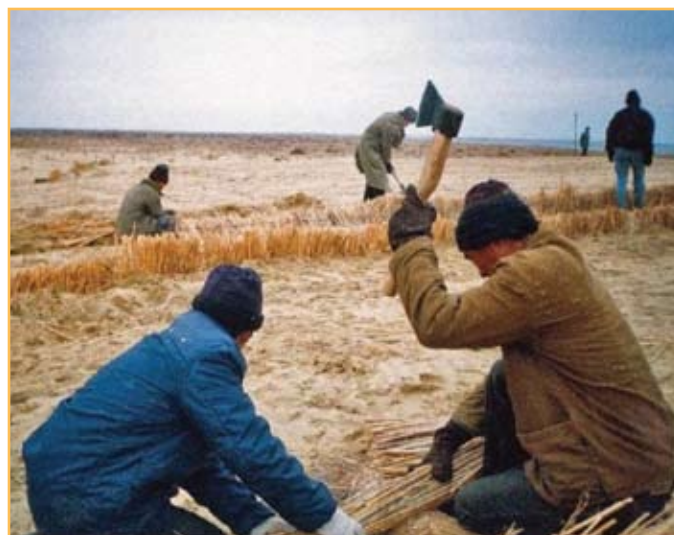
Creating sand protection belt around a village in Kazakhstan.
