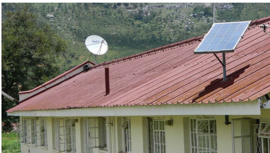
A rural health facility with installed VSAT powered by solar panel.
