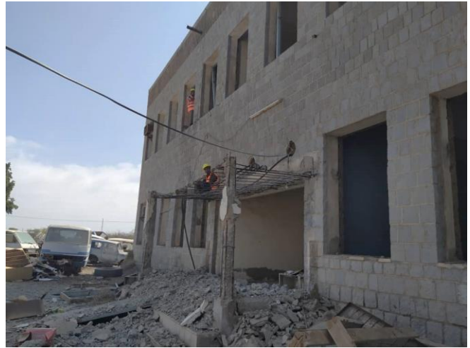
Rehabilitation of training center in the port of Hodeidah
