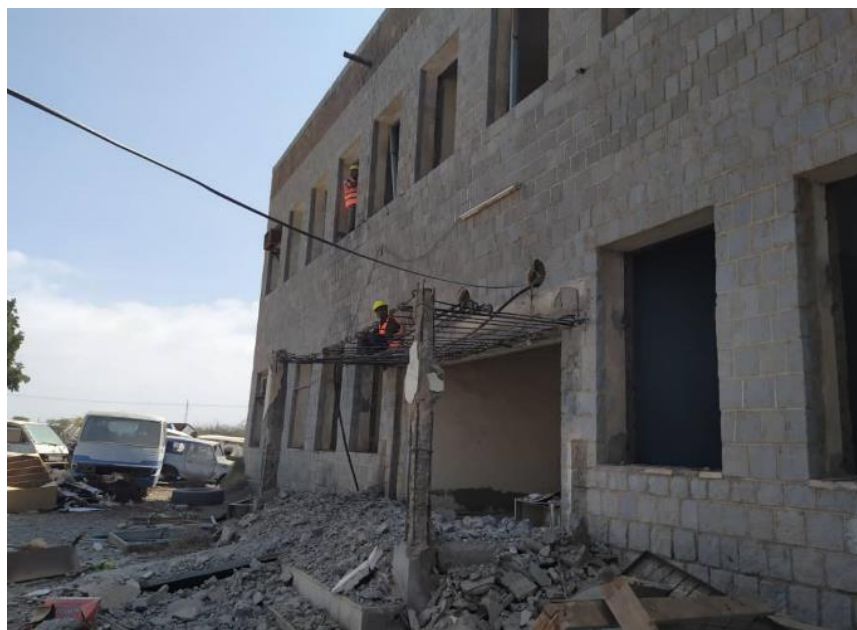
Training Center at Port of Hodeidah (under rehabilitation) – September 2019.
