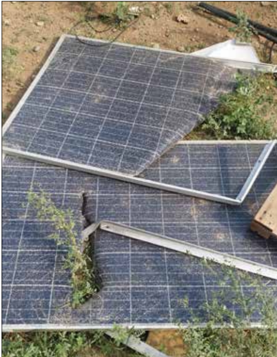
Al Khashm Health Unit, Al-Zuhrah District, Hodeidah (Photo Credit: AFCAR)
