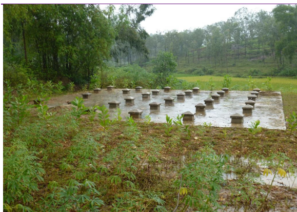
Figure 3.1 The bunker at Nui Cang
