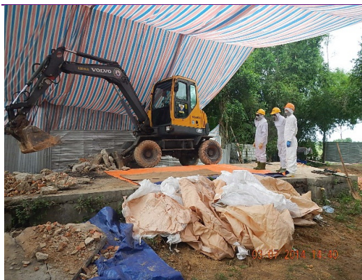
Figure 4.11 The excavation of the contaminated soil from the bunker
