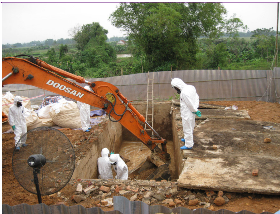
Figure 4.12 The excavation of the contaminated soil from the bunker
