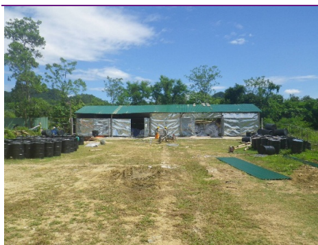
Figure 4.10 The big bags were stored in a neighbouring warehouse
