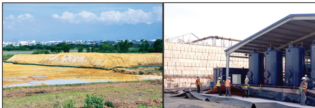
Figure II.14: Dioxin treatment at Da Nang airport
