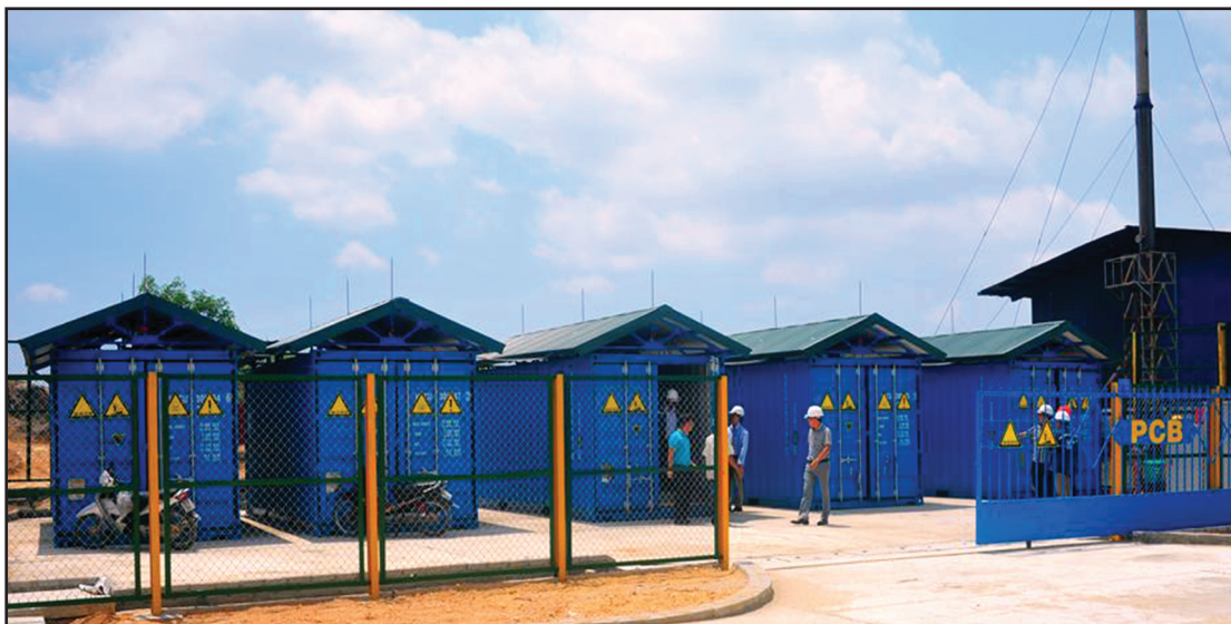
Figure II.12: Creating PCB waste storage in the form of containers
