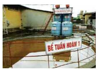
Figure 4: Construction of settling tank for pulp recovery and pulpy water circulation
