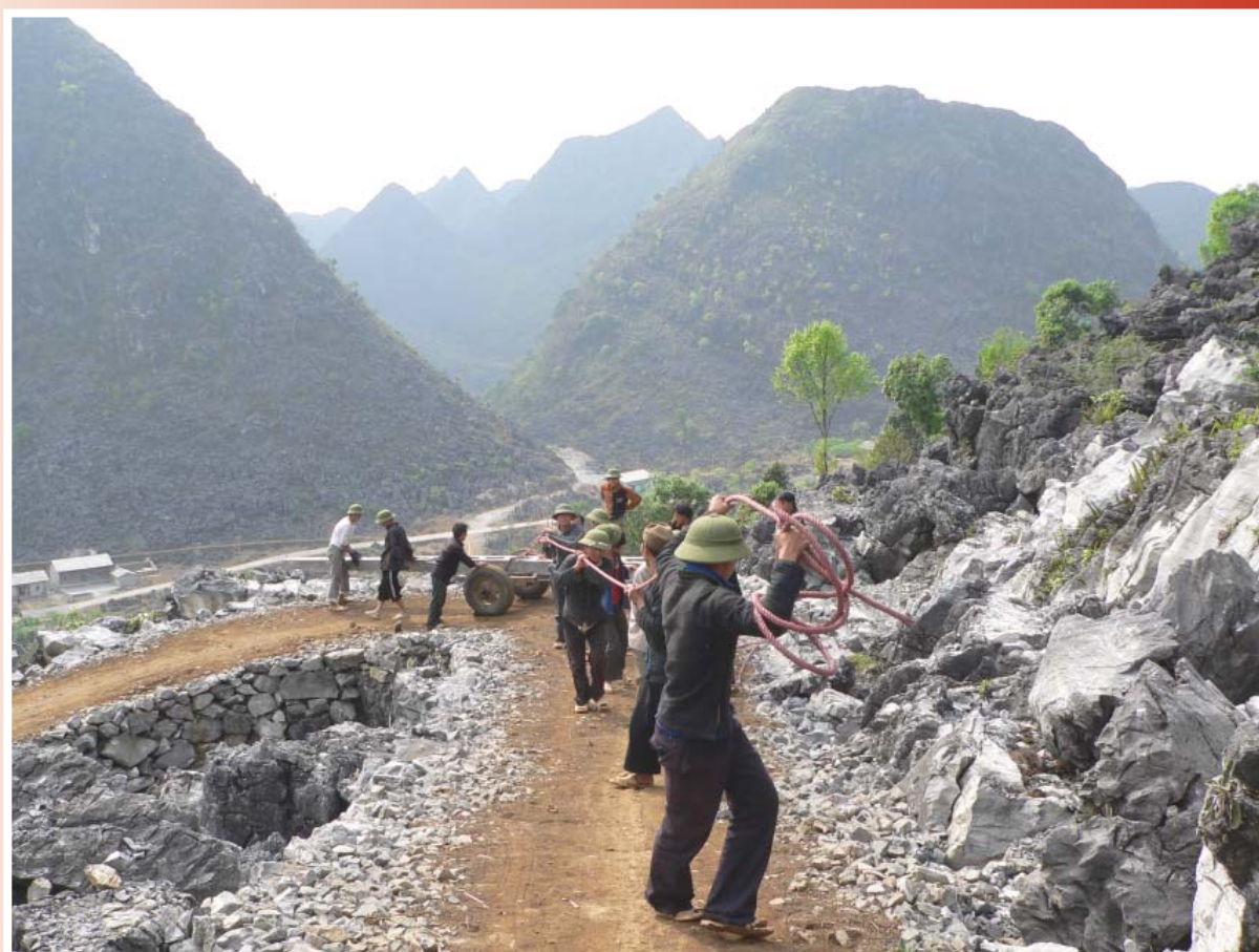
"Electricity Infrastructure Improvement" , Photo: Kiều Vân
