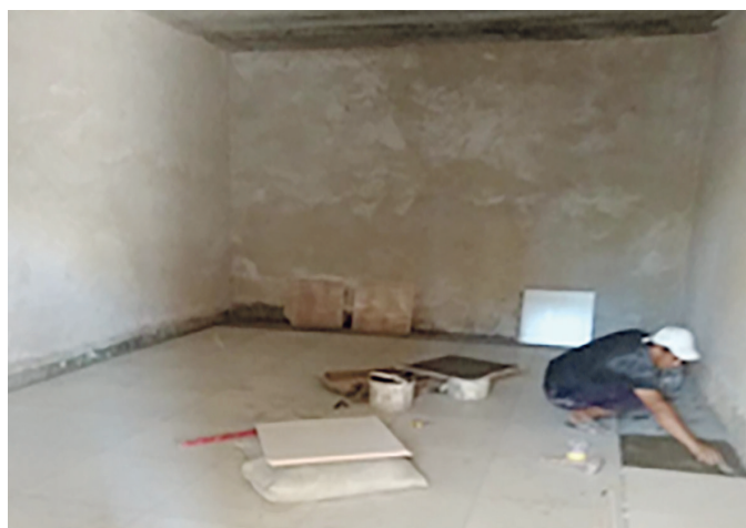
Pic.9. Reconstruction works at "SEYT SHARWA" farm.
