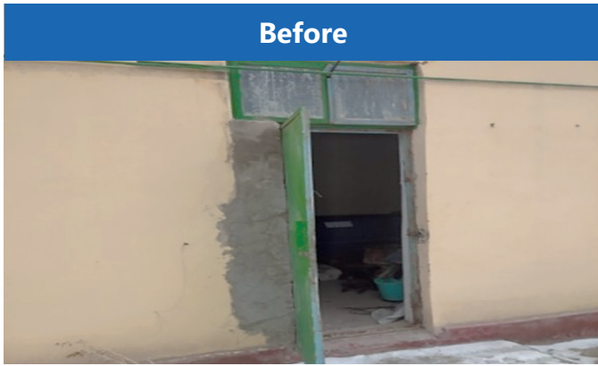
Pic.23. Building that was reconstructed for the workshop.
