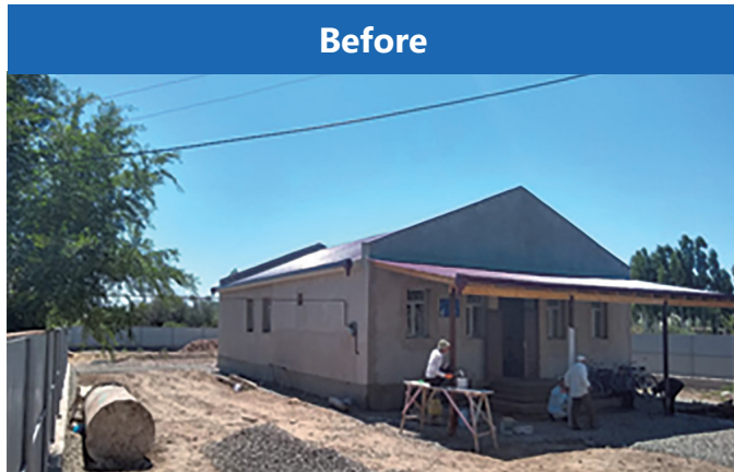
Pic.7. Reconstruction works at "SEYT SHARWA" farm.
