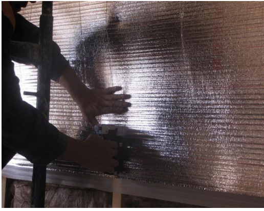
Attachment of the Isocom vapor barrier film
