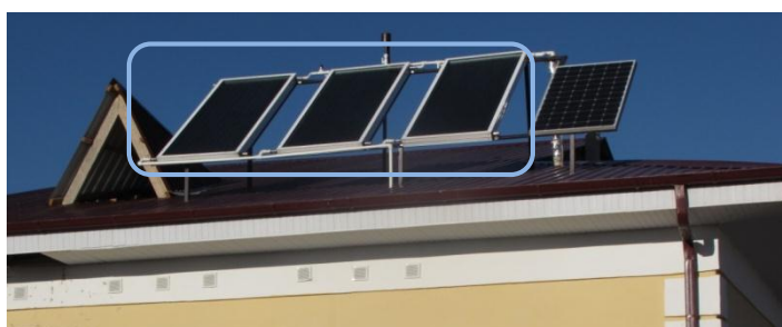
Figure 2.1.7. Solar water-heating collectors for hot water supply of the pilot rural house
