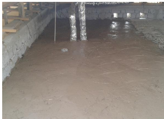
Insulation of the attic floor
