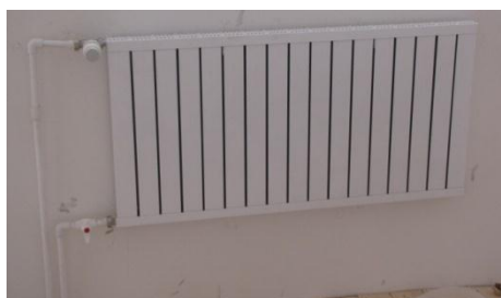
Figure 2.1.4. Aluminum sectioned radiators
