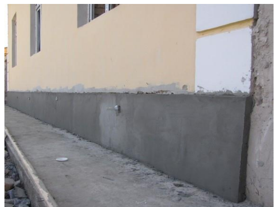
Insulation of the foundation at the base of walls
