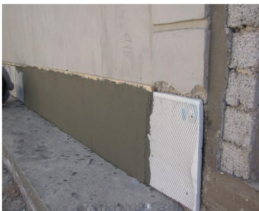
Insulation of the foundation at the base of walls
