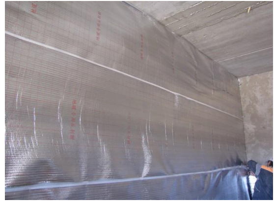
Attachment of the Isocom vapor barrier film
