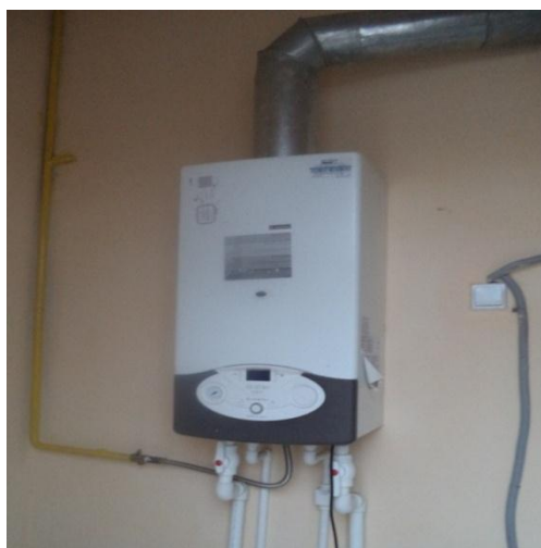
Figure 2.1.3. Gas-fired wall-mounted single-contour automated Ariston boiler
