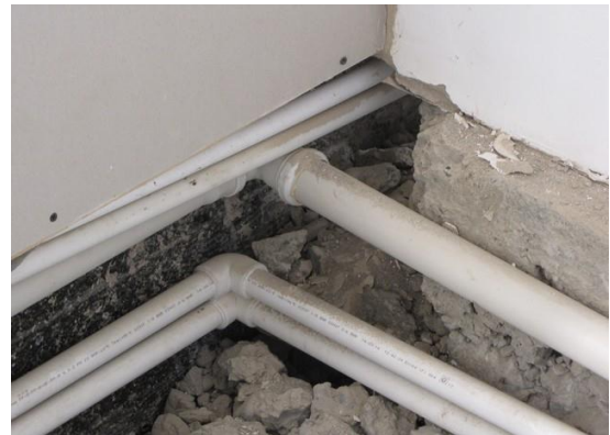
Two-pipe heating system
