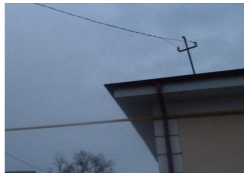
Entry point for electricity
