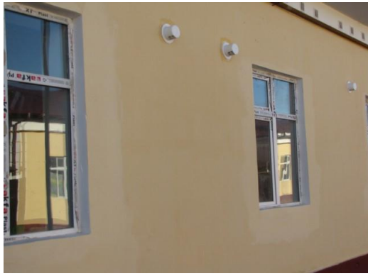
Wall-mounted heat recovery ventilators
