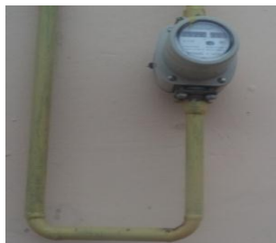
Figure 2.1.6. Gas meter
