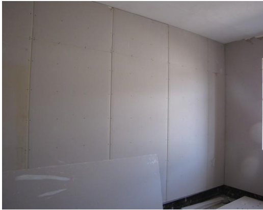
Plasterboard paneling
