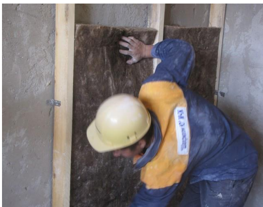
Insulation (from inside the house)
