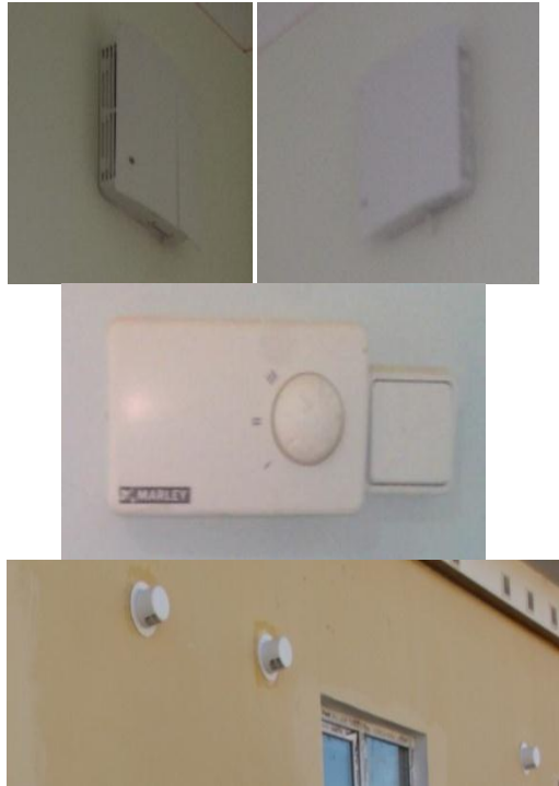
Figure 2.1.8. Heat recovery ventilators of the house
