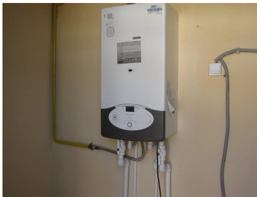
Wall-mounted autonomous boiler
