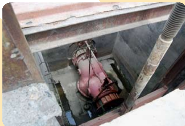
A turbine of a microhydro power station that Rustam Tashmatov independently established in the Zavrak village.
