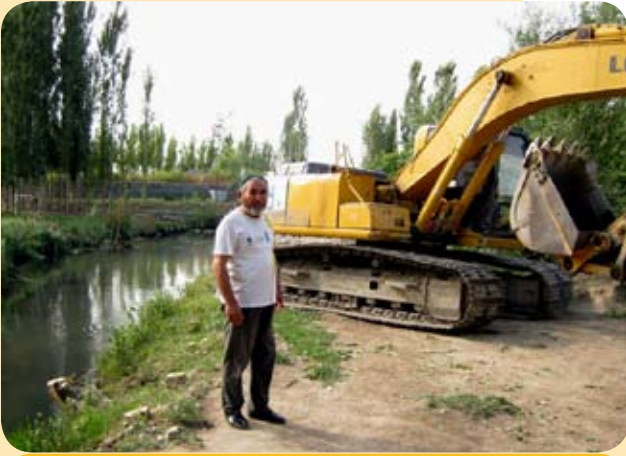
Rahmatullo Shodiev and the excavation works.
