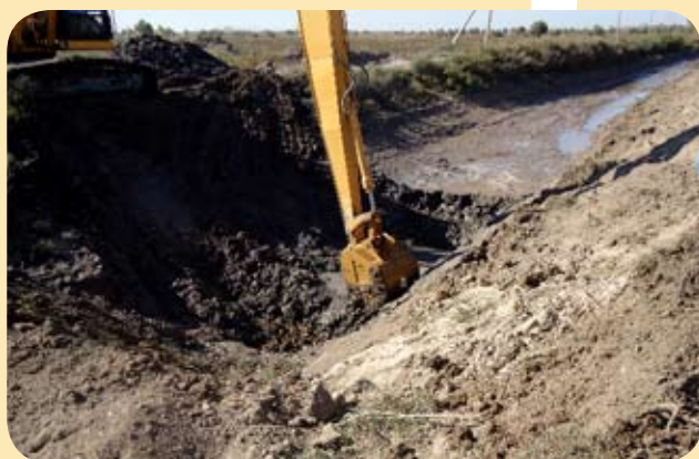
Excavating works on cleaning and preparing works of 'Navruz-yap' canal.
