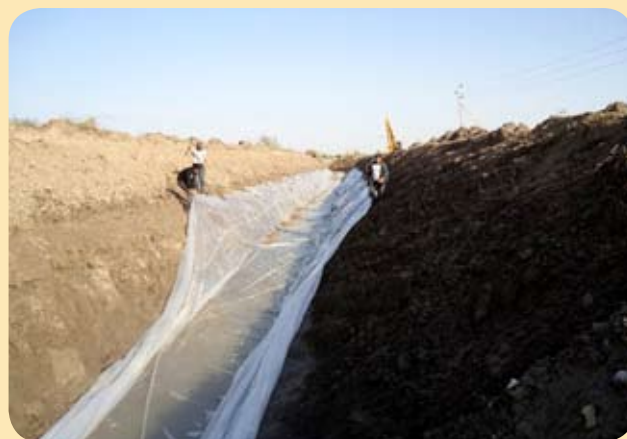
Arranging an isolated tape at the bottom of the canal.
