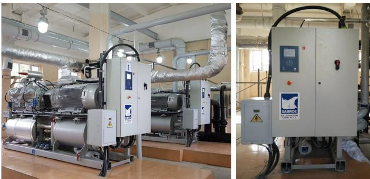
Figure 9. General view of the new chiller running on R717.
