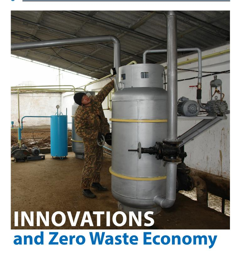
Global Environmental Facility Small Grants Program (GEF SGP) has helped launch a biogas facility in the 'Ulugbeklar' farm located in the Turakurgan District, Namangan Region. Its reactor capacity is 100 cubic meters which is well enough to generate biogas and heat food. Beyond meeting the farm's needs, Mahmudjon Kodirov, the head of the farm, is planning to supply free biogas to school #8 in the nearby village 'Yangi Kishlok'.
