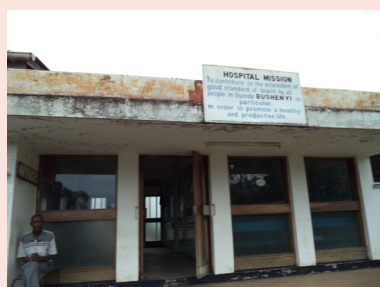
Kitagata hospital - Main Block
