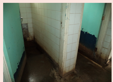
Kitagata hospital- Bathrooms in Maternity ward
