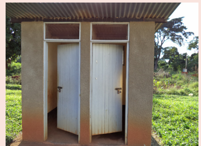
Toilets at Kigandalo HCIV-Mayuge
