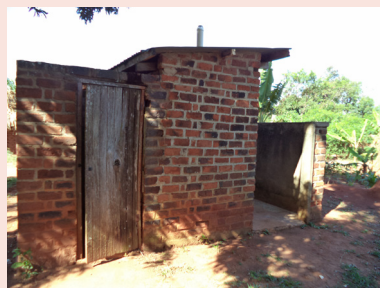
Toilet for Malongo HCIII-Mayuge
