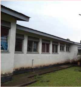
Kitagata hospital-The very old hospital structures
