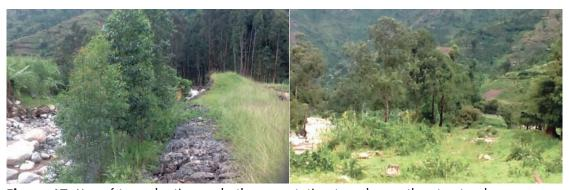
Figure 17: Use of tree planting and other vegetation to enhance the structural measure
