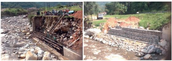
Figure 14: Re-construction of wall at the bridge near Nyamwamba sub-county and roll stone protecting
