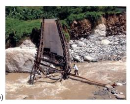
Figure 10: (a) Part of the River bank [see white arrow, near Bulembia primary School] that over flowed causing flooding in Kilembe town. Note the deposition of boulders in the channel on the right. (b) Destroyed bridge following blockage of flow by large boulders
