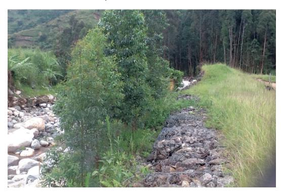
**Figure 13:** Embankment enhanced by tree planting on R. Nyamwamba, upper Kilembe Town,
