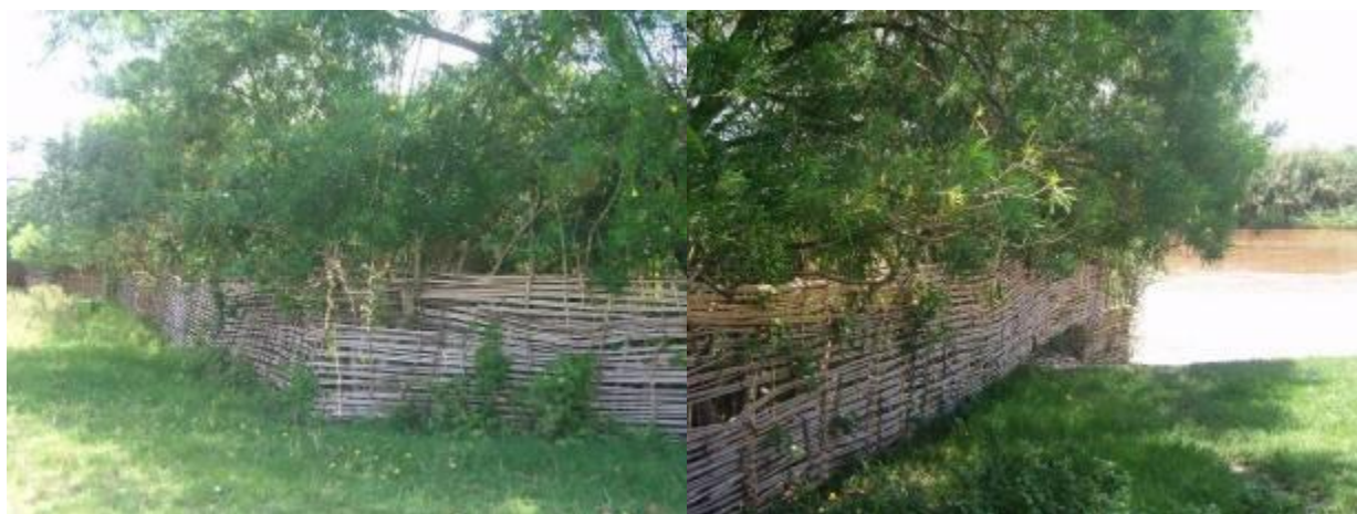
Plate 12: Fencing to control erosion and flooding on Semliki River
