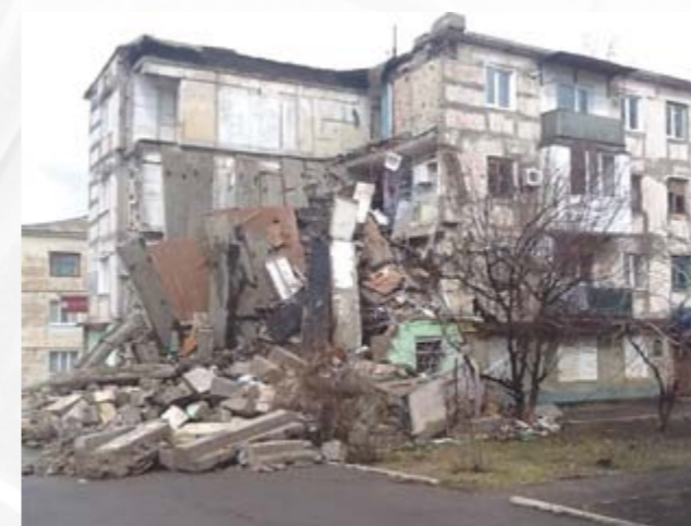
Destroyed house in Pervomaysk 2
