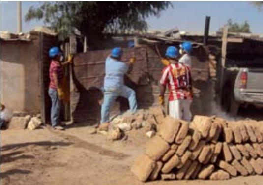
Removal of recycled PCB-containing materials used as building material in a community of San Felipe Nuevo Mercurio
