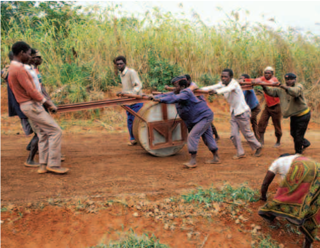
Construction of a rural road using a hand-operated roller near Lugela, Mozambique, 2001 (Neil Cooper/Panos Pictures)
