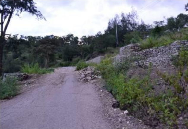
Figura 9 – Evidencia husi Inundasaun be suli habelar, Rai-halai no erosaun, no esforsu enjineria atu proteze strada
