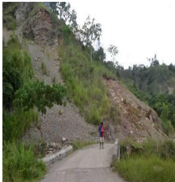
Figura 8 – Rai-halai taka Estrada no fo ameasa ba ponte, kauza husi rai-lolo, la konsolida ho fatuk, fini vegetasaun. Suco Baguia, Kaptasaun Boro Uai
