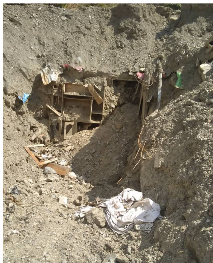
Figure 43: Houses destroyed due to the land slides
