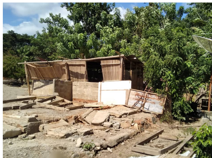
Figure 42: Miscellaneous (wood, CGI sheets, bamboo) debris
