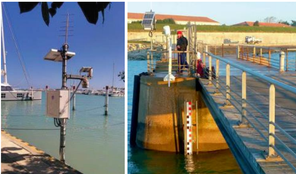
Figure 15. Site photos of instrumental setup in the Caribbean (left) and France (right) to obtain water level variations. From these images we see radar gauges, with accompanying power source (solar panels). From the Caribbean setup the box containing the data logger and shown set off the ground as well as the communication antenna. From the France example, in addition to the radar gauge (the white instrument mounted on the concrete wharf pylon) an example of tide staff or tide board is shown.
