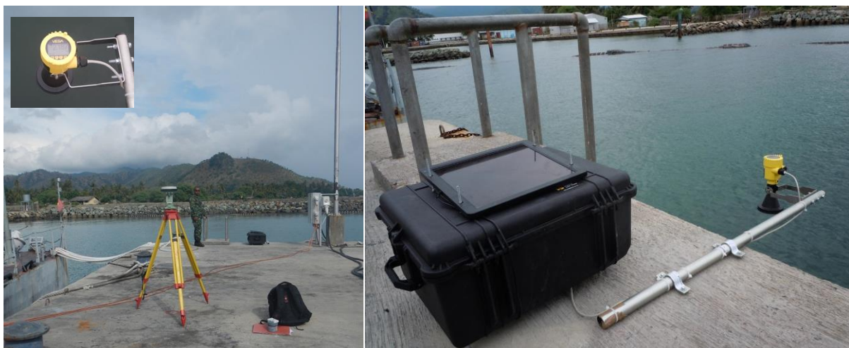
Figure 10. Site photos of the Orinoco Vega Plus Radar tide gauge at the Hera Naval Base. This instrument is equipped with a Vegaplus 61 sensor (inset photo). These images were sourced from the Relatorio Technico Dos Trabalhos De Campo 2014 Report. From the instruments shown in the right panel, it appears care was taken to survey the elevation of radar gauge sensor so that data from the gauge could be accurately referenced to a land benchmark.
