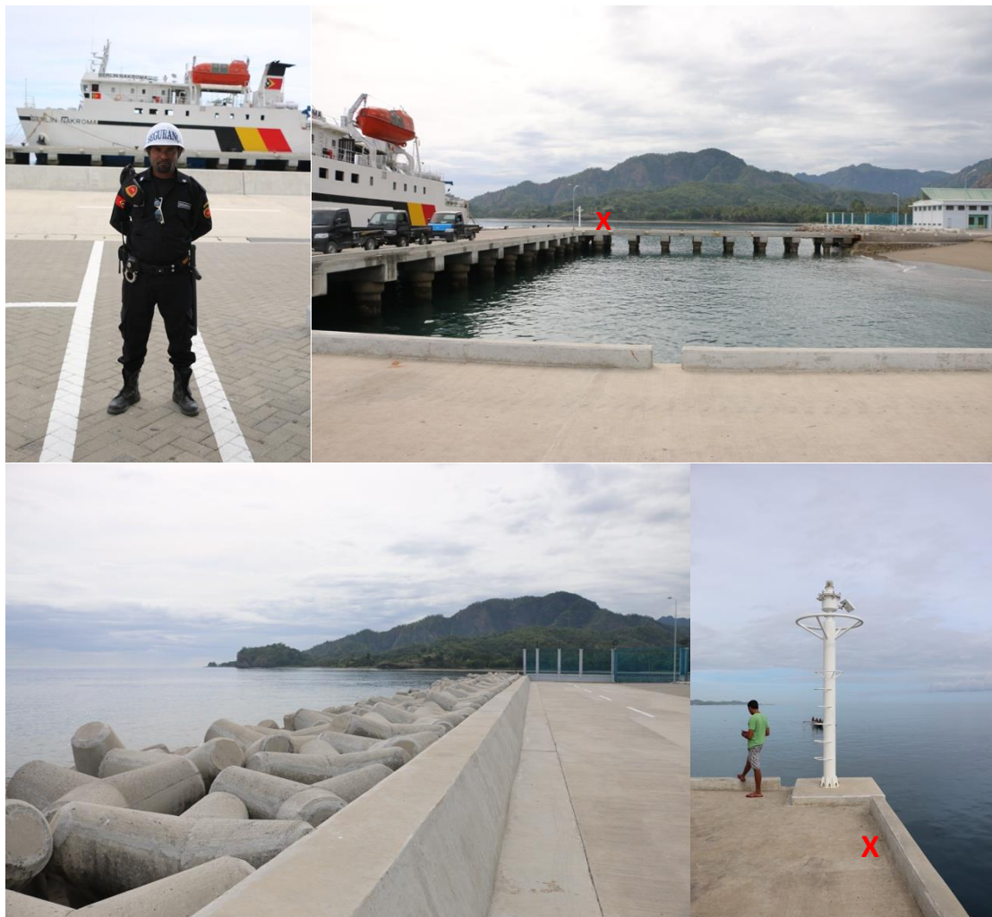
Figure 12. Site photos of Mahata Port, taken during the rapid coastal assessment 10 th April – 5 th May, 2017. The red X indicates the proposed location of tide and sea level instruments. Large concrete shapes called tetrapods are used to protect some sections of the port from waves.
