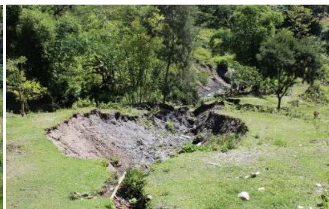
Figure 24 – Gully erosion on sparsely vegetated pasture. Mertutu Suco, Lois River Catchment
