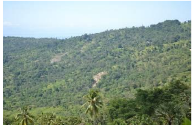
Figure 10 – Example of moderate slope and sparse vegetation contributing to the risk of landslides. Abafala Suco, Uai Muhi Catchment
