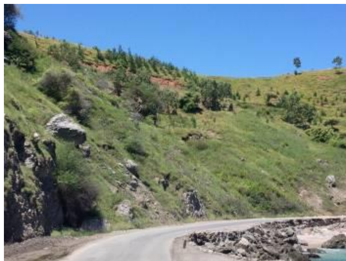
Figure 30 --Stabilization efforts with tree-planting on landslide-prone slope. Ulmera Suco, Comluli Aggregate Catchment
