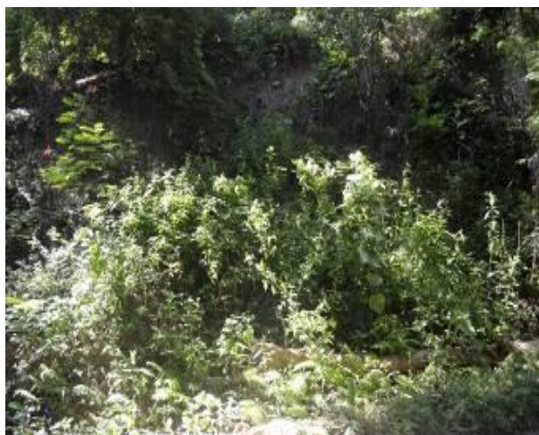
Figure 1 – Roadside landslide. Buruma Suco, Baucau Aggregate Catchment
