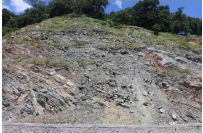
Figure 43 – Severe erosion on steep slope with thin, friable soils and no vegetative cover. Vatuboro Suco, Sanakiana Aggregate Catchment
