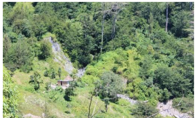
Figure 20 – The nature of Ermera landslides – small, isolated, right next to a house. Poetete
