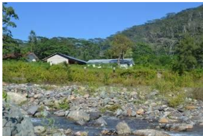
Figure 16 – School and health post threatened by river erosion and flooding. Mertutu Suco, Lois River Catchment
