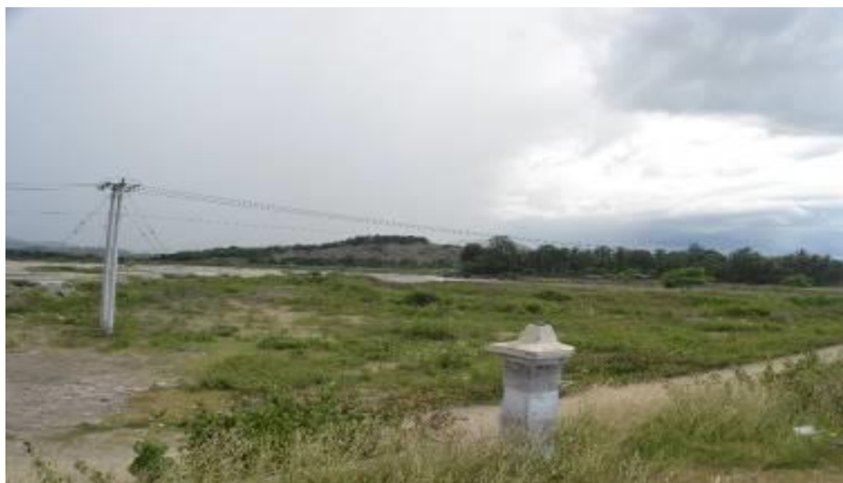
Figure 13 – Regular flooding threatens roads and electricity infrastructure. Vemassee Suco, lower Vemassee River Catchment
