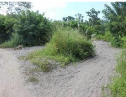
Figure 37 – Road in flood zone. Suco Guico
