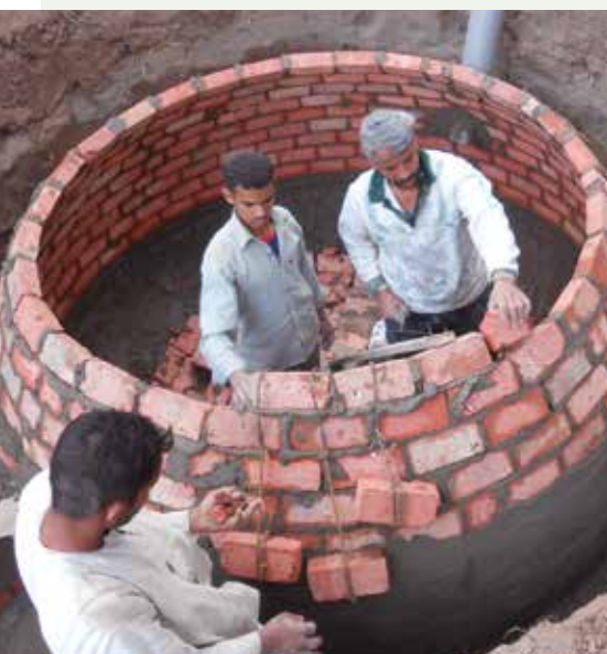
Installation of biogas digesters for household energy needs in Egypt. Photo by UNDP Egypt
