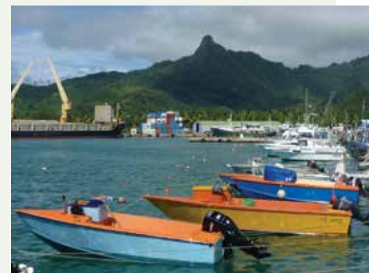
Climate proofing coastal infrastructure in the Cook Islands. Photo by Celine Dyer and Robert Matapo
