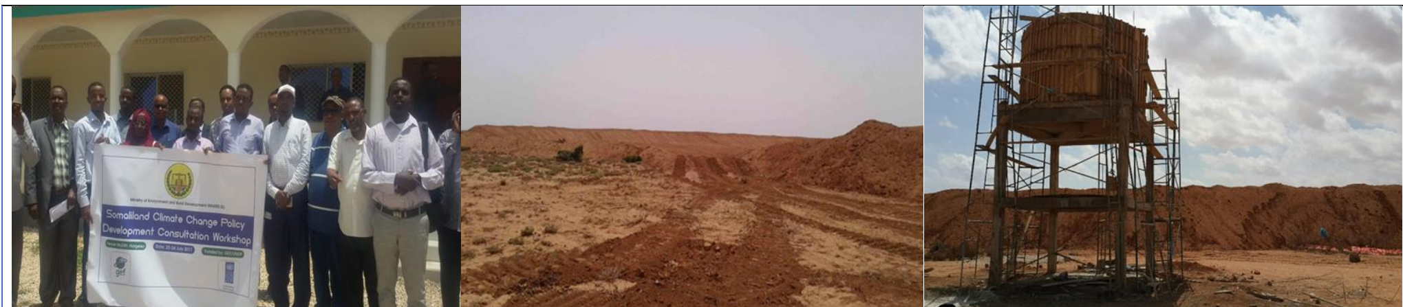
Figure 5: Photos Showing Somaliland Climate Change Policy Consultation Workshop and Construction Stages for Baligubadle Earth Dam in Somaliland
