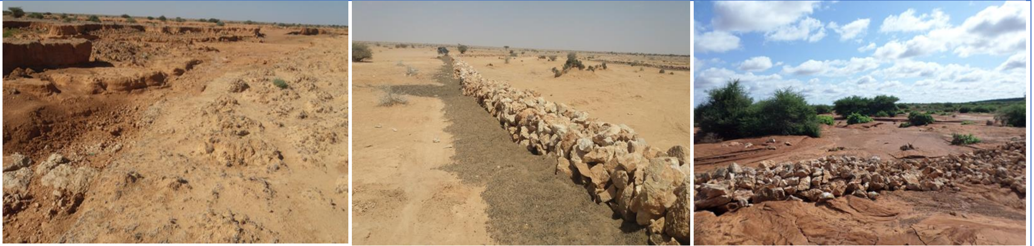
Figure 1: Before and After Photos of Balidacar Water Diversion in Garowe District of Puntland Region
