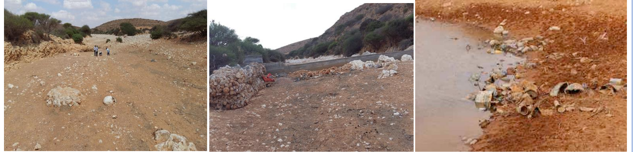
Figure 2: Before and After Photos of Dangoryo Dam in Puntland Region
