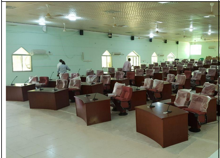
Refurbishment of the Puntland House of Representatives
