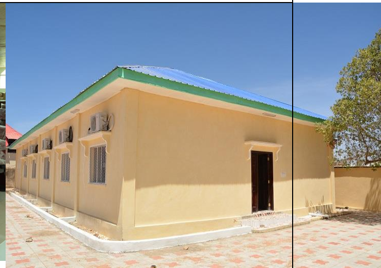
Construction of South West State Assembly Secretariat Office Building
