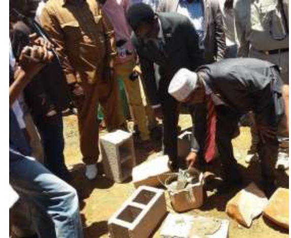
Initiation of ISWA Multi-Purpose Facility Construction – Baidoa
