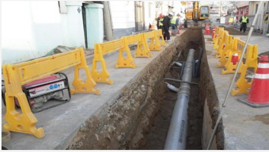
Sewer pipe under construction (BTL program) 50
