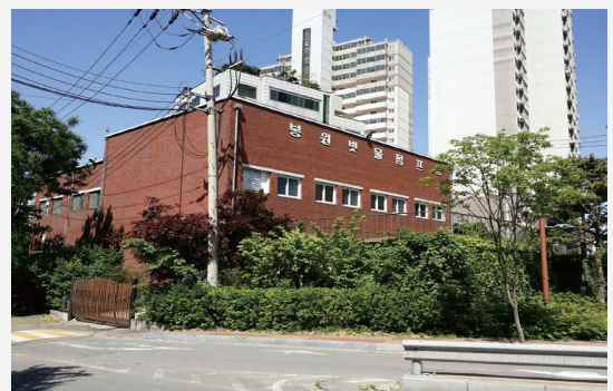
Storm Water Pumping Station in Seoul
