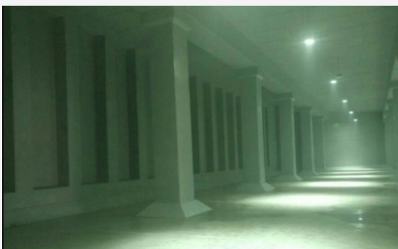
Storm water storage facility in Seoul
