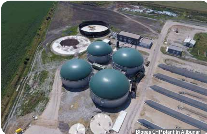
Biogas CHP plant in Alibunar
