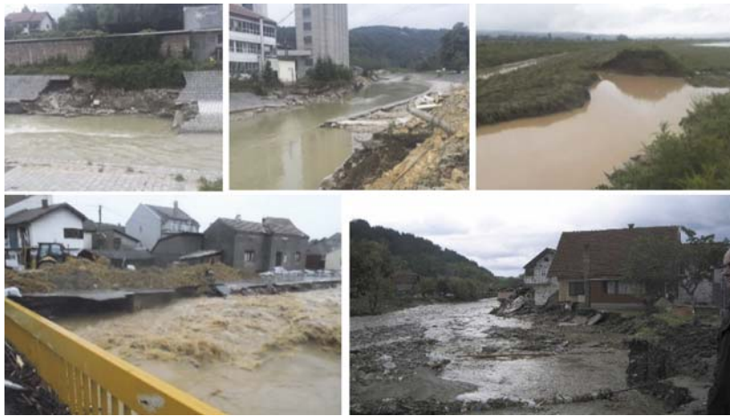
Picture 2: Destroyed and Damaged Water Management Infrastructure
