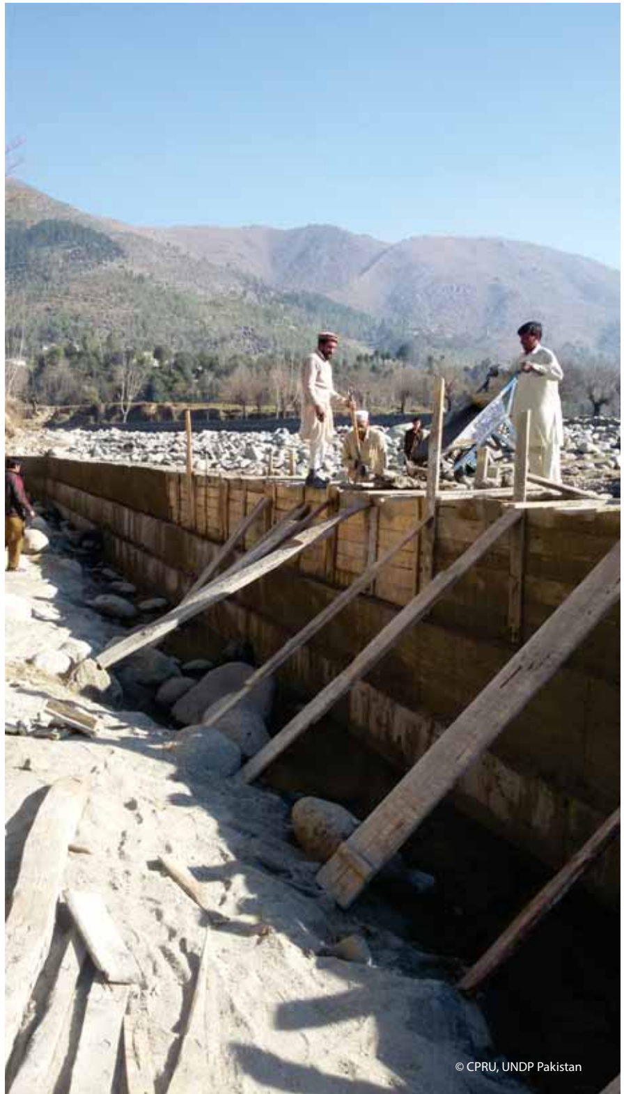
Flood protection wall being constructed in Kotky Shahi Khel, Lower Dir
