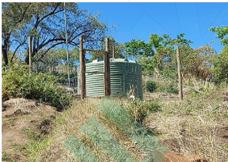
Fenced water tank area located at project site, Ba, Fiji (Photo by MRMDDM)
