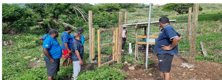
Tuvu settlement residents inspect water infrastructure, Ba, Fiji (Photo by MRMDDM)
