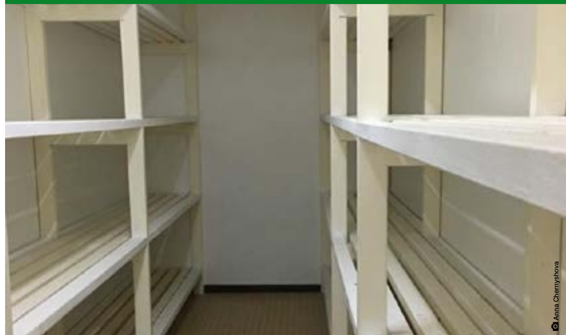
A view from inside the newly renovated National Bednet Storage Center.
