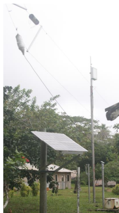
Three Generations of Dysfunctional Communications Infrastructure at Sarawia Disp: Solar-powered HF Radio, TVL public telephone and solar-panels to charge mobile phones (neither working) leave no options for emergency communication
