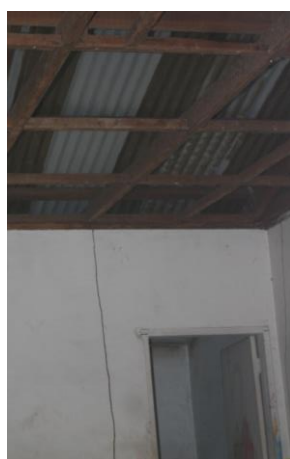
Damaged ceilings and walls to inpatient ward at Bemisas HC
