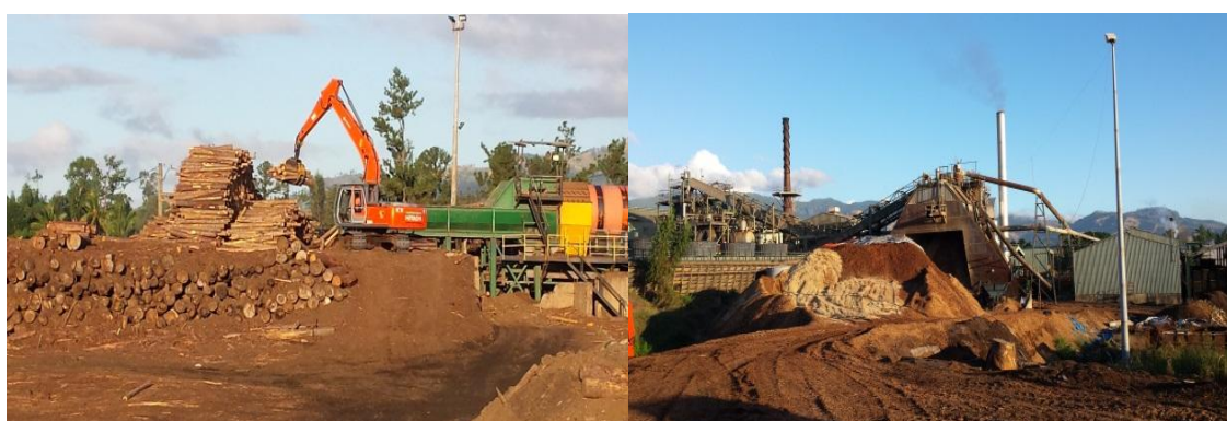
Figure 6: TWIL Biomass Waste Power Plant at Drasa (Source: TWIL)
