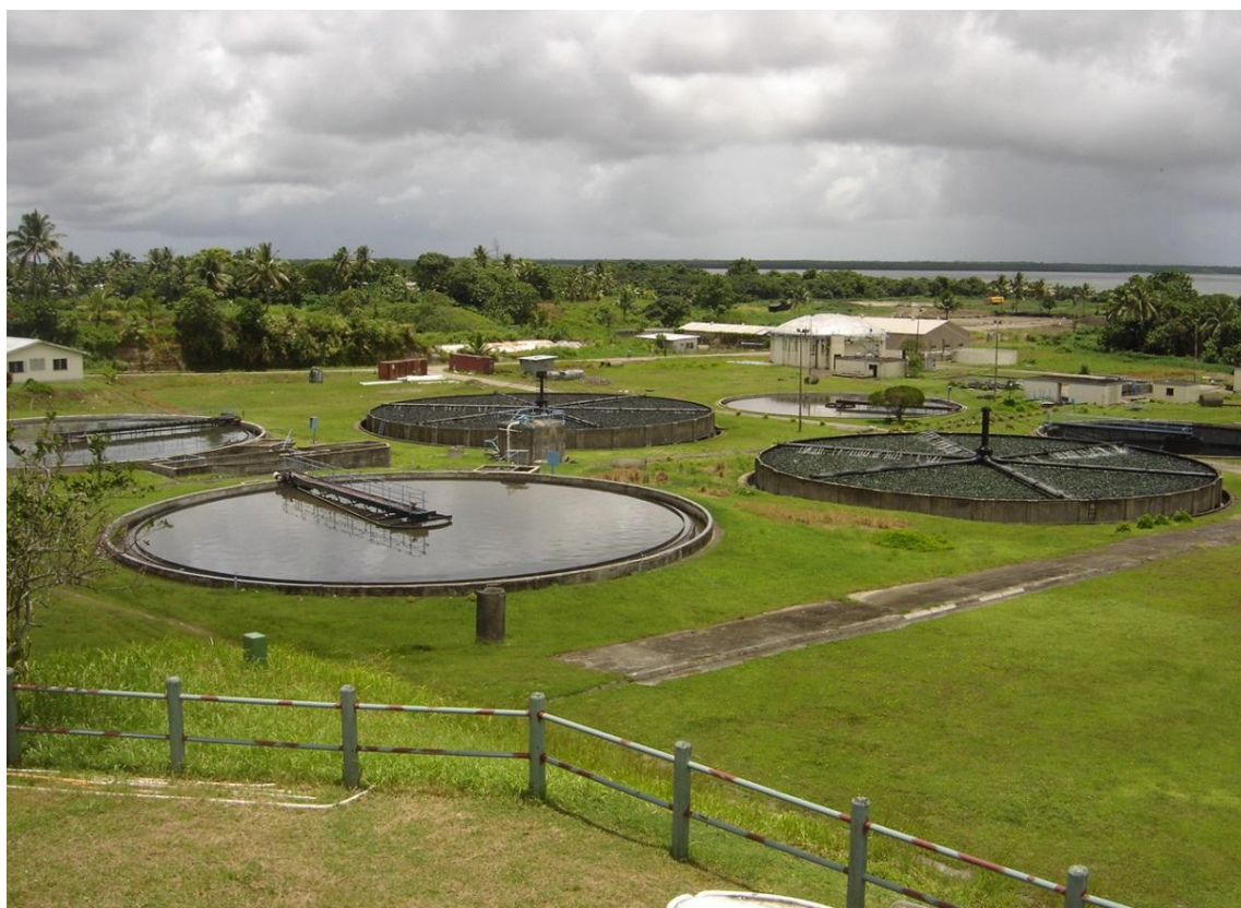
Figure 5: Kinoya Sewage Treatment Plant, Suva-Nausori (Source: WAF)
