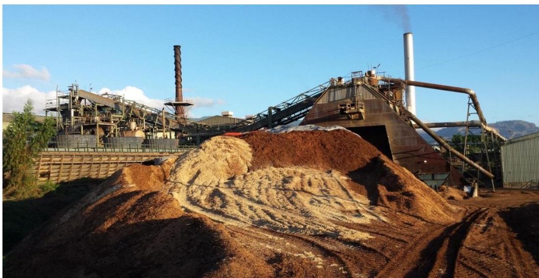
Figure 13: TWIL Biomass Waste Power Plant at Drasa (Source: TWIL)
