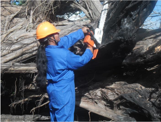
Debris removal, 'Uiha, Ha'apai.
