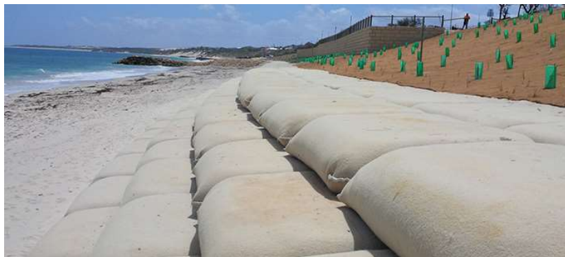
Figure 17: Example of back of beach geo-textile revetments
