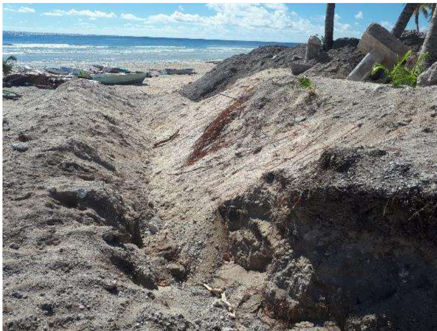
Figure 54: Construction works on Nanumaga beach surrounding the church foundations in 2018
