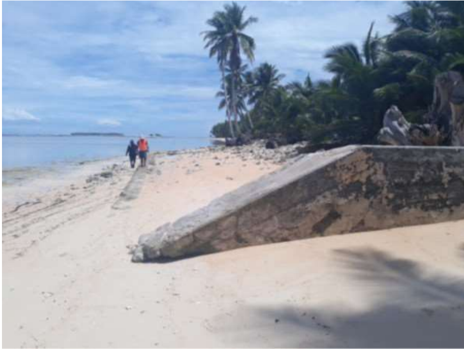
Figure 11: Existing Nanumea seawall with foundations and wingwall remaining
