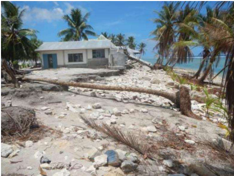
Figure 33: House undermined and eroded on Nanumea
