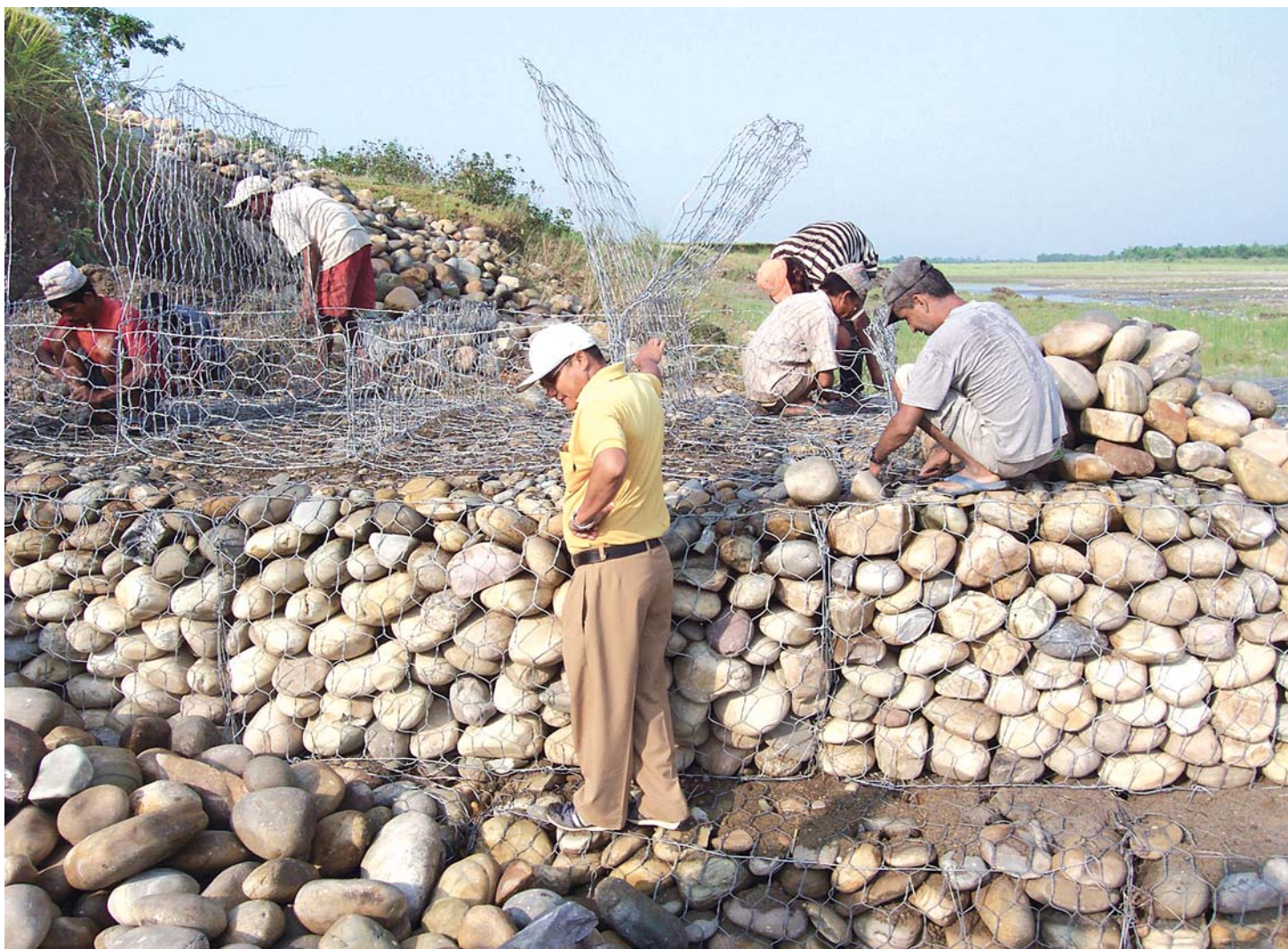
Local people of Gardi village in Chitwan district constructing embankment using stones and gabion wires
