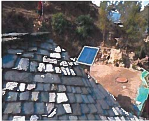
Solar Home System (21 WP) installed with the support from NCCSP, Achham district
