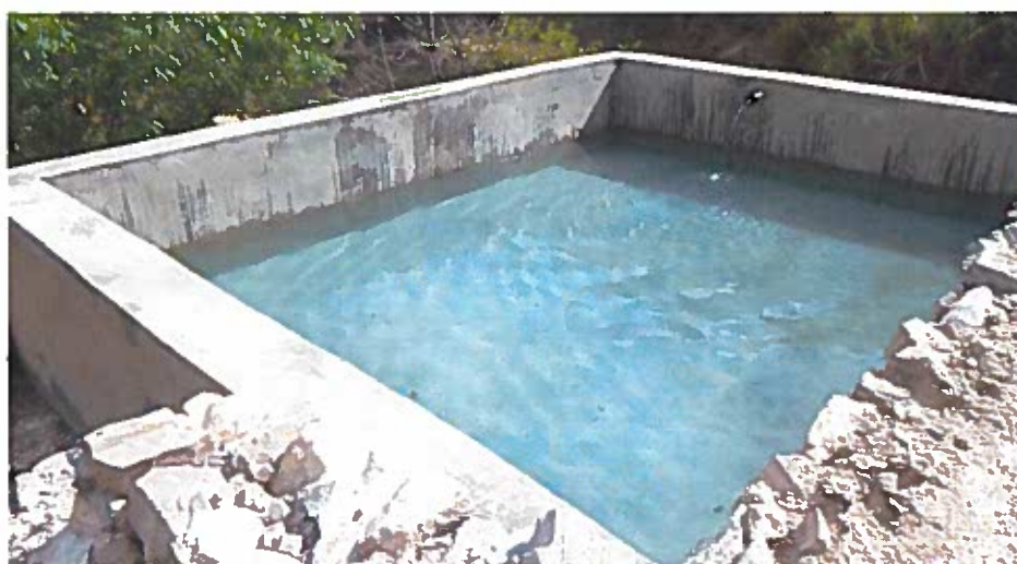
Picture 6: Chalabang Irrigation Pond in Gaam VDC, Rolpa
