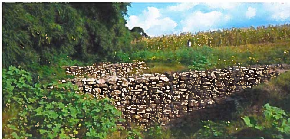
Gabion wall, Bela VDC, Dang
