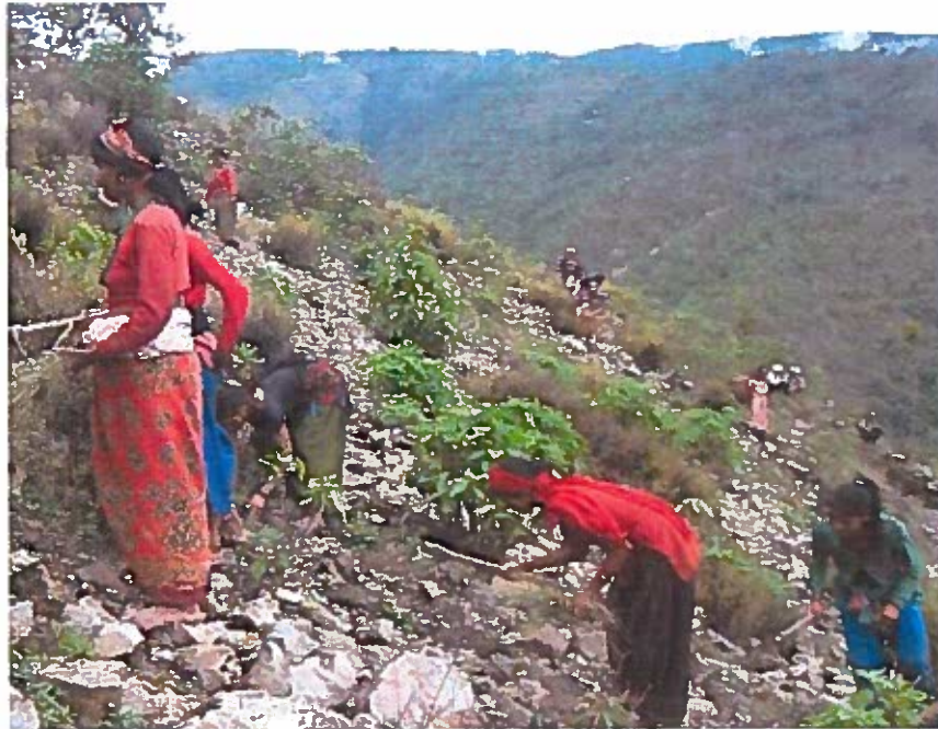
Picture 4: Slope stabilization through Plantation, Dailekh
