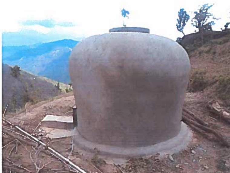
Picture 2: A rainwater harvesting tank, built in Dullu, Dailekh
