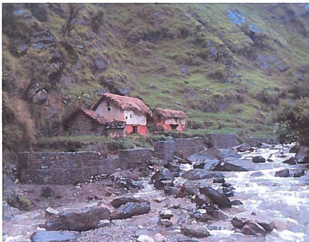
Picture 6: Gabion wall constructed in Lohare River, Kalika VDC, Dailekh
