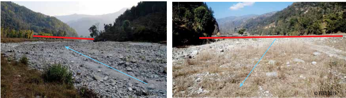
FIGURE 27: PROPOSED SILTATION DAM LOCATION AT KHAHARE KHOLA OPTION 1 (LEFT) AND OPTION 2 (RIGHT)
