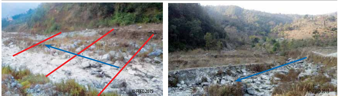
FIGURE 29: GENERAL VIEW OF BETENI KHOLA AND LOCATION OF CHECK DAMS
