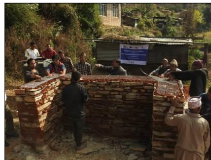
(e) Another example of participants installing WWM bands
