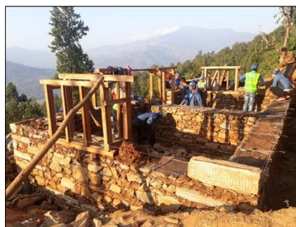
(b) Installation of window frames
