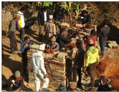
(b) Participants installing cross-links
