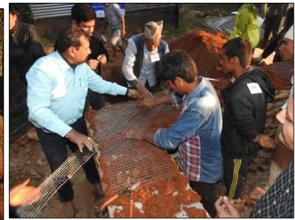
(c) Participants installing WWM bands
