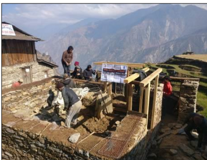
(a) Installation of WWM band
