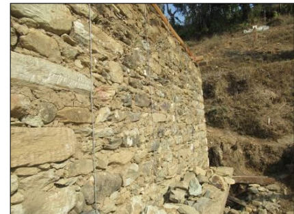
(c) Close up view of vertical wires
