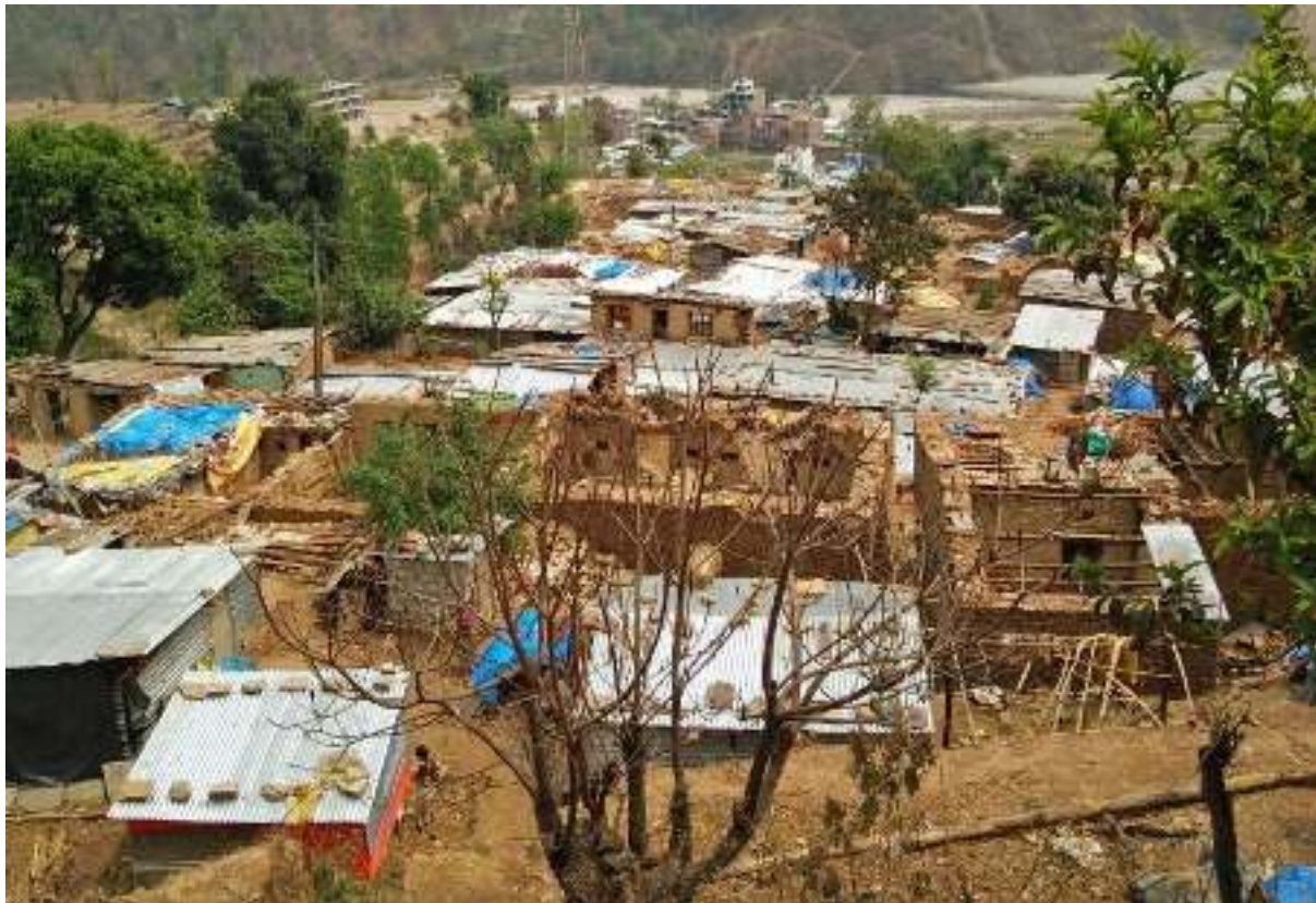
Post-earthquake slum-ification of Thulaghar and Digaun in Majhigaon
