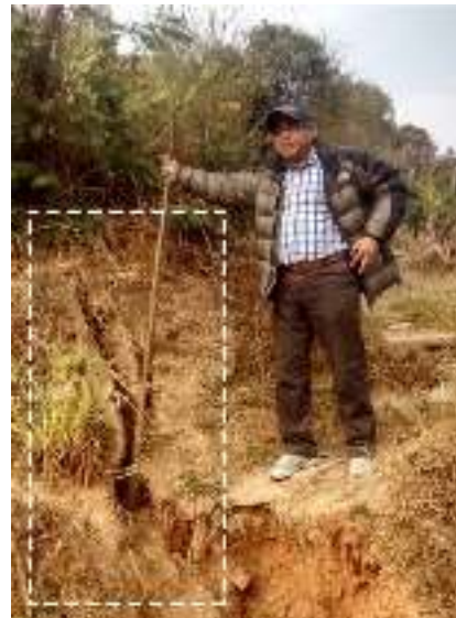
Prof. Ajay Lal showing crack in Majhi Gaon
