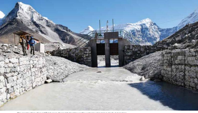
The construction of an artificial open channel helped lower the water level in Imja Lake by 3.4 metres.
