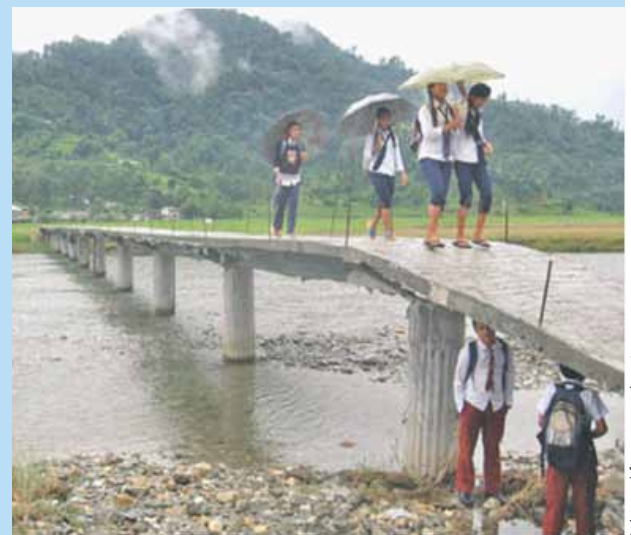
Student crossing the newly built trail bridge
