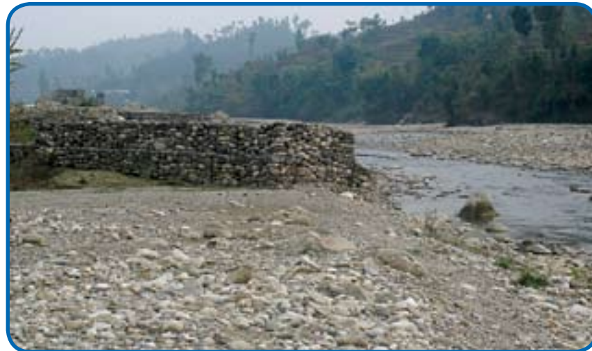
Gabion spur in Ambhanganj VDC, Hetauda
