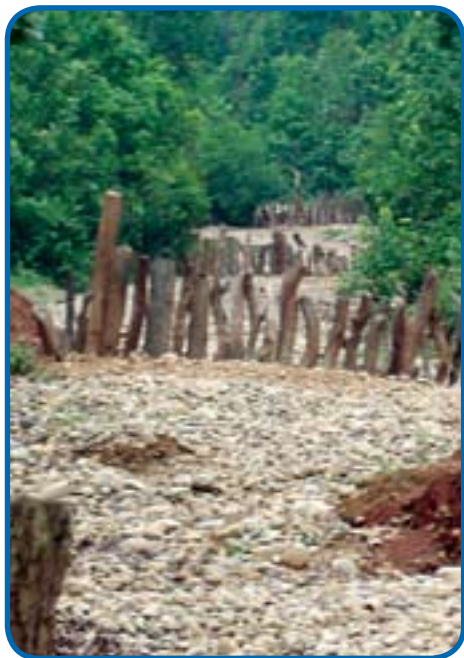
Series of wooden check dams to control debris flow in Nepane VDC, Sindhuli
