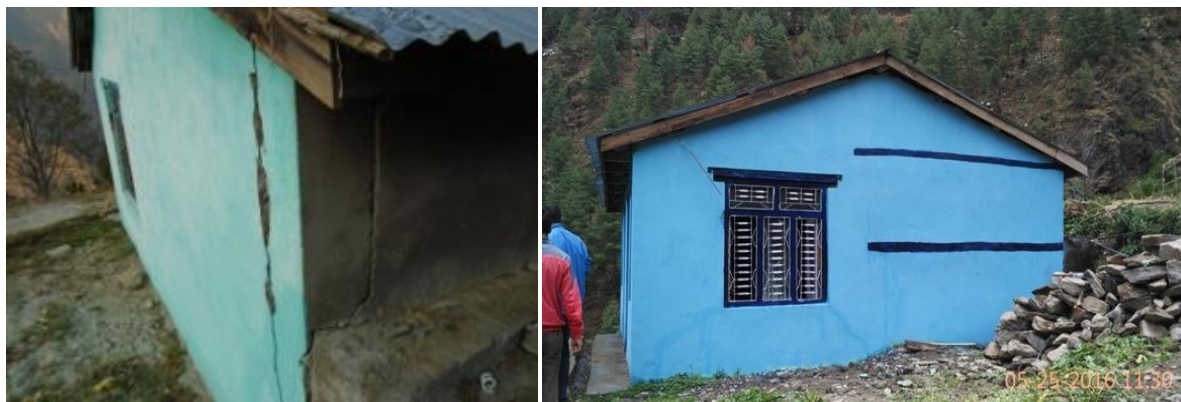
A repaired CFC in Rasuwa
