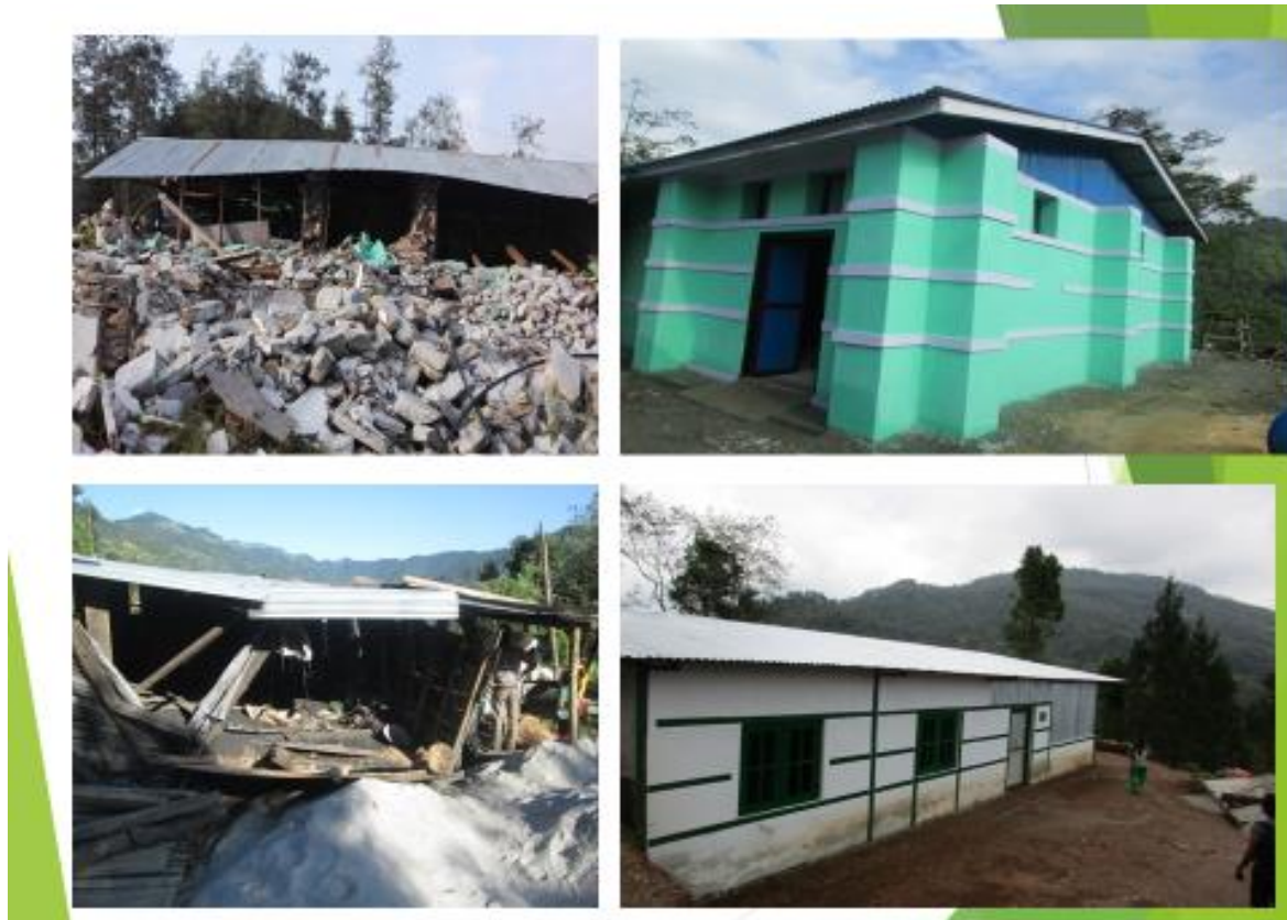
Rebuilt CFCs in Sindhupalchowk
