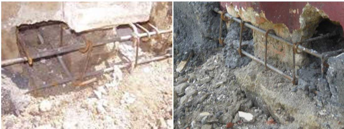
Figure B-8: Retrofitting works for the tie beam (inserting tie beam)
