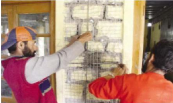
Figure A- 9: Tying encasement reinforcement to bear connector dowel
