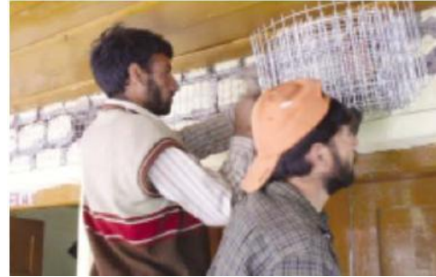
Figure A- 8: Installing WW mesh from aroll
