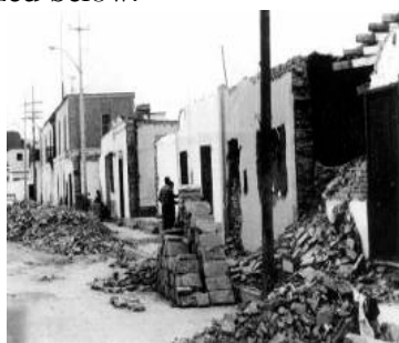
Figure 2.1 Severe damage to adobe buildings in Chorrillos district in Peru earthquake 1974 (Source: www.earthquake.usgs.gov )
