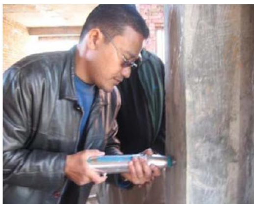
Fig A.I. 1.(a)Use of Rebound Hammer
