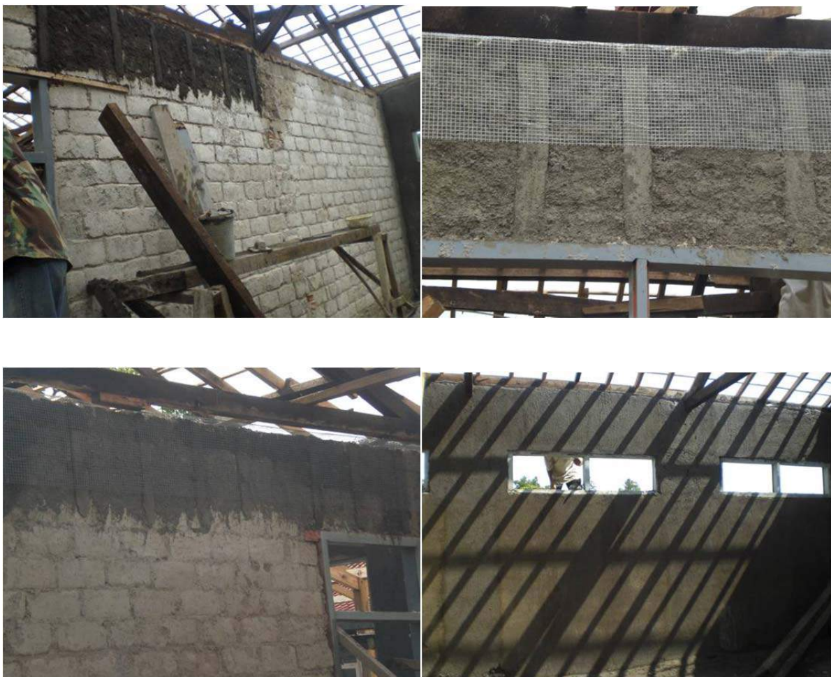
Figure B-10: Retrofitting works for the wall (cont'd)
