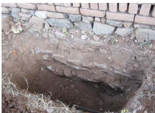
Exploration of foundation
