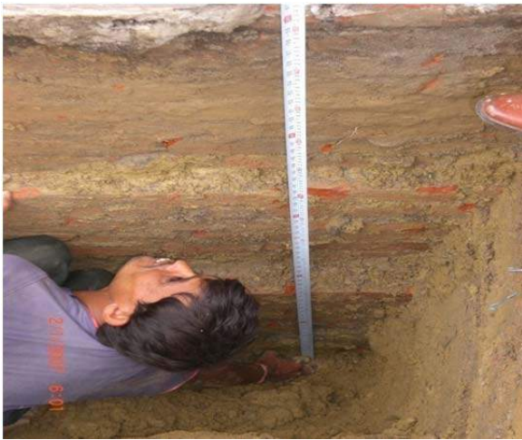
Figure B-17: Foundation Exploration
