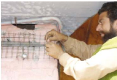
Figure A- 13: Installing 'L' shaped dowel at corner to ensure continuity
