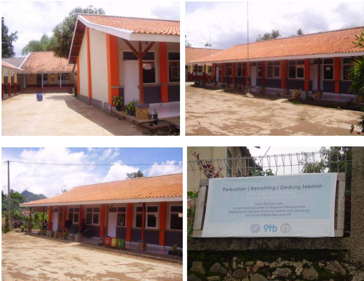
Figure B-14: Finishing works (painting, architectural gravel installation, etc)
