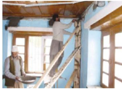
Figure A- 16: Vertical reinforcement concreting formwork
