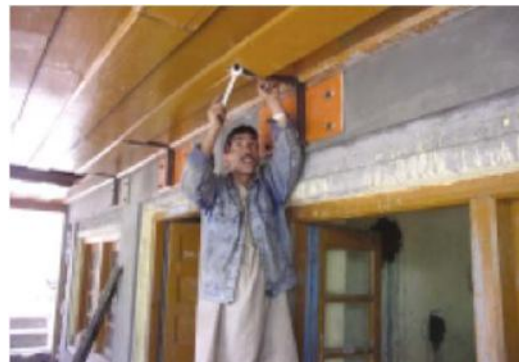
Figure A- 19: Installing bolts and brackets for roof-wall connection
