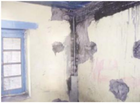
Figure A- 15: Installing vertical reinforcement in the corner
