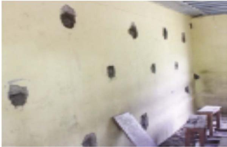
Figure A- 4: Bond elements yet to be completed in RR wall
