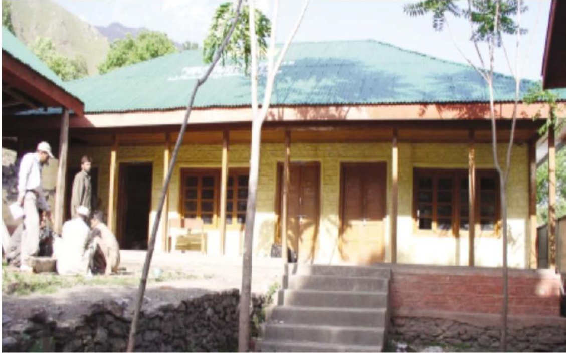
Figure A- 2: Existing 3 room school building before retrofitting
