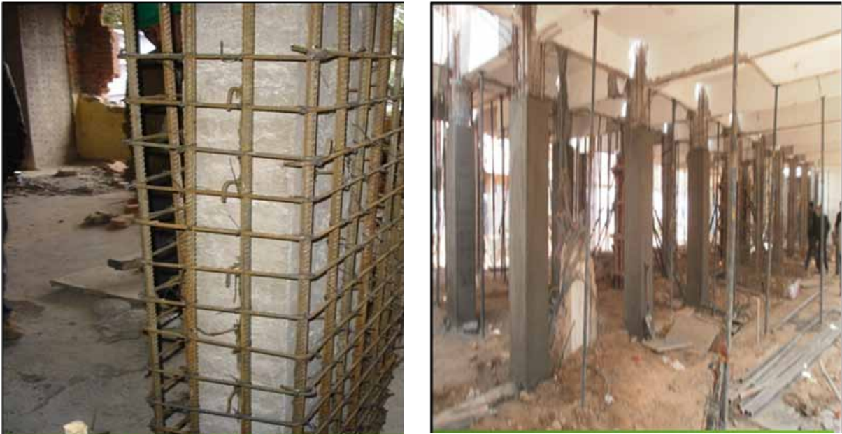
Figure 6.8 Jacketing of column (source MRB & Associates)
