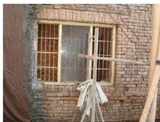
Fig A. I. 4(c) Wall Jacketing in process
