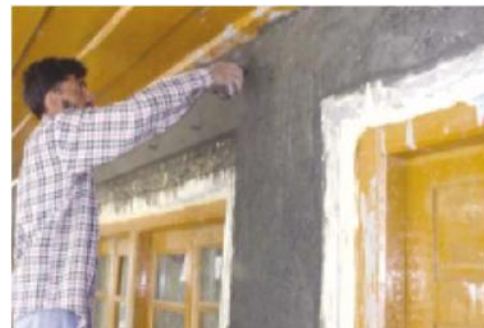
Figure A- 14: plying cement-sand plaster
