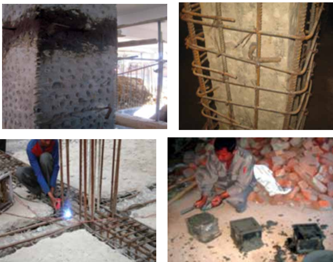
Figure 6.6 Strengthening of original structure (Source: MRB & Associates)
