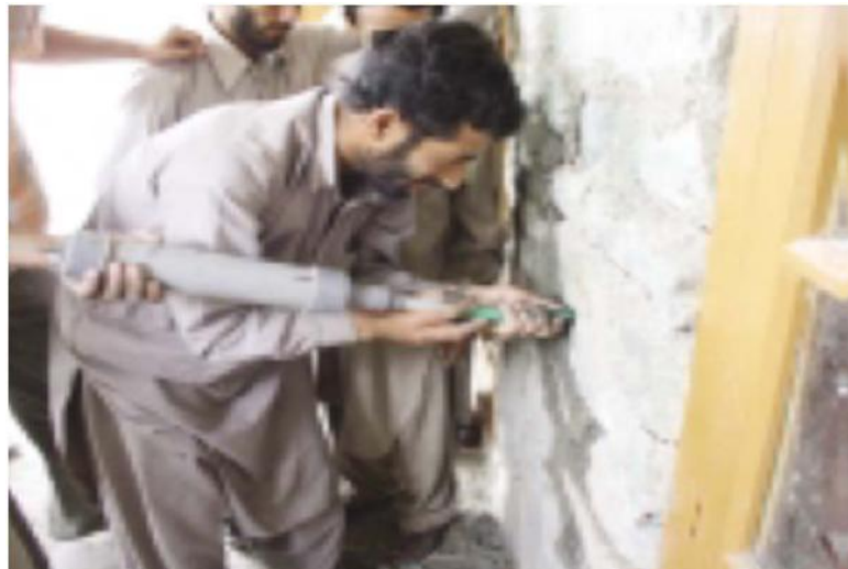
Figure A- 5: Grouting no-shrink grout in crack with hand pump
