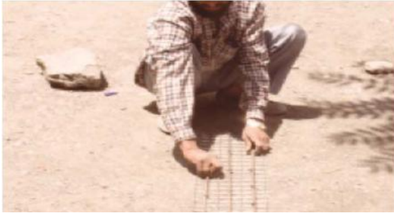
Figure A- 7: Preparing WWM with 6 mm rebars
