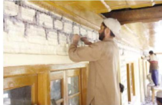
Figure A- 10: Installing belt reinforcement
