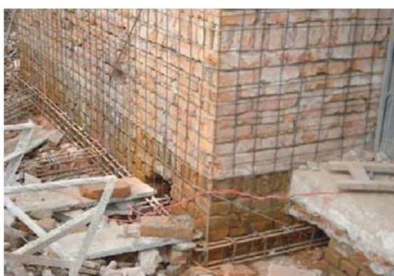
Fig A.I.4(b) Erection of Reinforcement for wall
