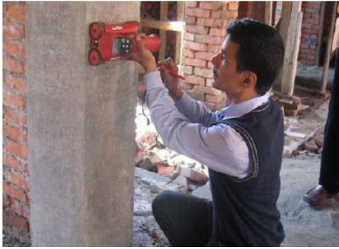
Fig A.I.2.(a) Use of Rebar Detector for Verification of Reinforcement Details
