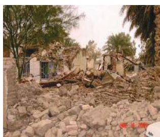
Figure 2.3 Collapsed adobe structures 2003 Bam Earthquake (Source: www.worldhousing.net/whereport1view.php?ID=100130 )
