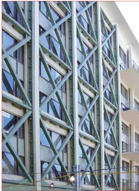
Figure 6.31 Addition of steel bracing
