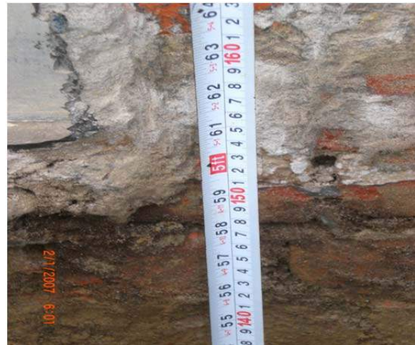
Figure B-18: Tie Beam Exploration
