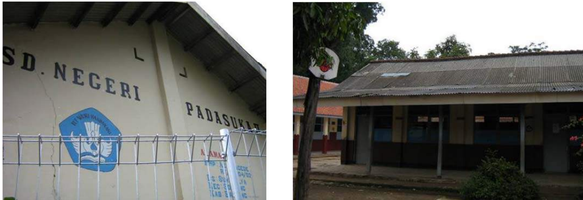
Figure B- 1: Layouts and Existing Conditions of SDN Padasuka II Prior to Retrofitting
