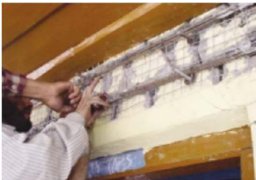
Figure A- 18: Installing bolts and brackets for roof-wall connection
