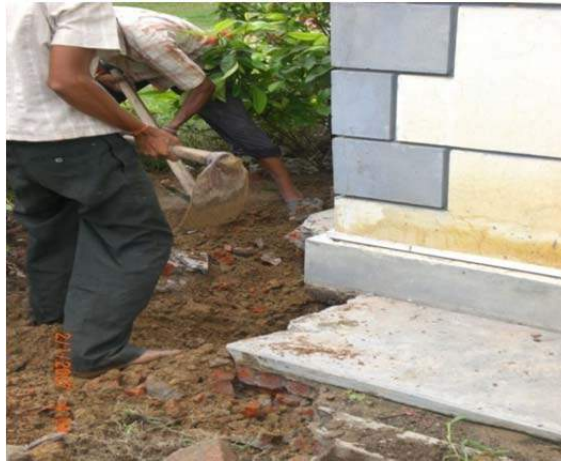
Figure B-16: Excavation for Foundation depth check
