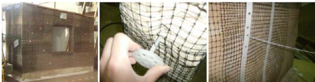
Figure 4.24 Reinforced house with geomesh
