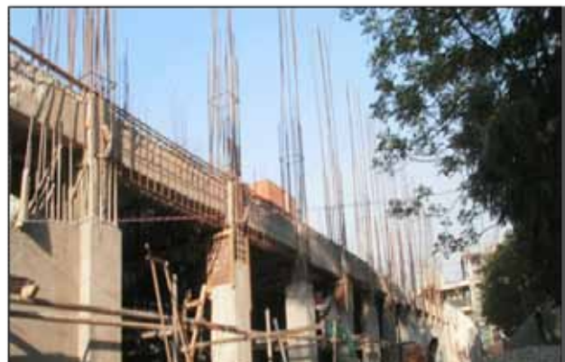
Figure 6.15 Encasement of existing beam (Source: MRB & Associates)
